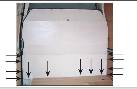
Carefully drill 4.5mm through the top sections fixing holes in the positions shown below and secure to the crossmember using No14x1/2" self tap screws (FX4087). (6 positions along the top and 1 position each side).
